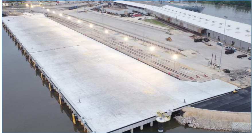
Beaumont's newly constructed Ro/Ro dock
