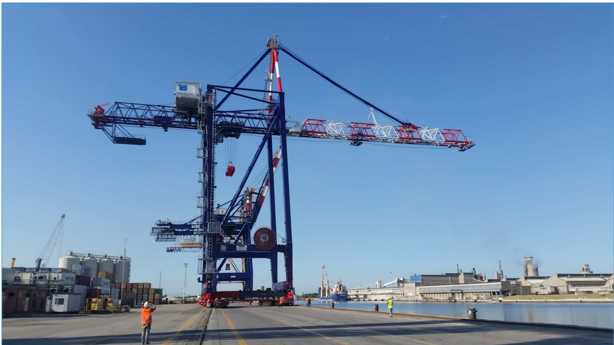
Ship-to-Shore gantry crane
